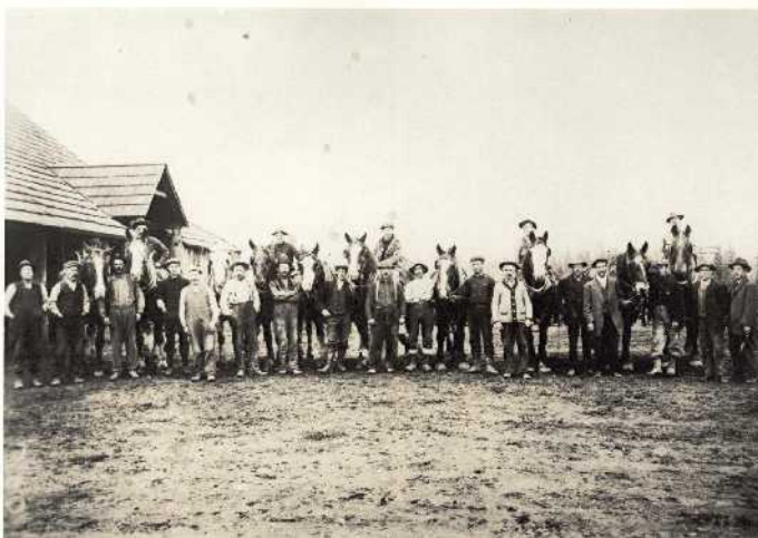
1912 Land clearing team Photograph from the Sydney Archives.
