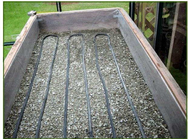
Heating cable laid over sand base
