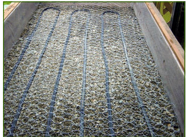
Layers of chicken wire laid over heating cable
